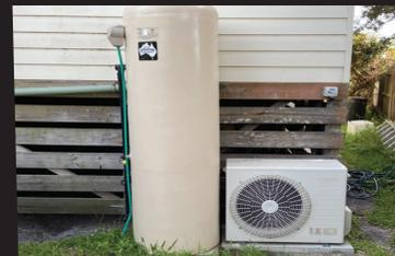
An electric heat pump hot water system will deliver hot water cleanly and efficiently.
